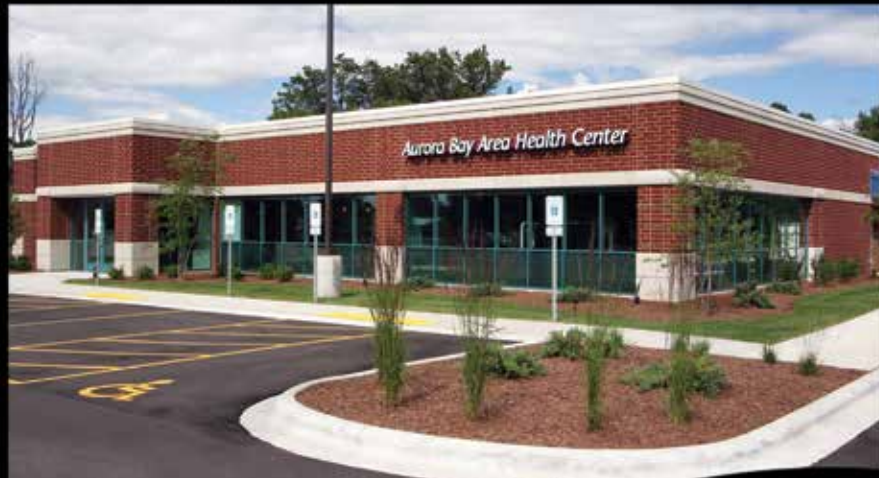
Build-to-Suit Health Care Facility Crivitz, WI
